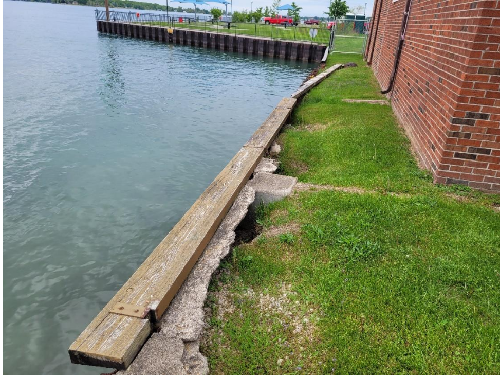
Washout/loss of backfill material
