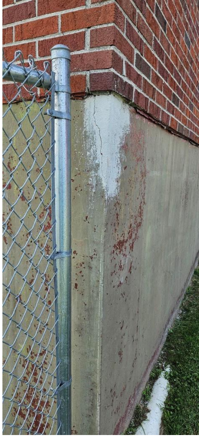
Cracking of exterior wall/foundation
