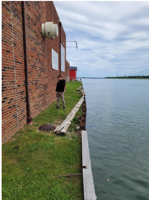
Bowed seawall and deteriorated/missing header
