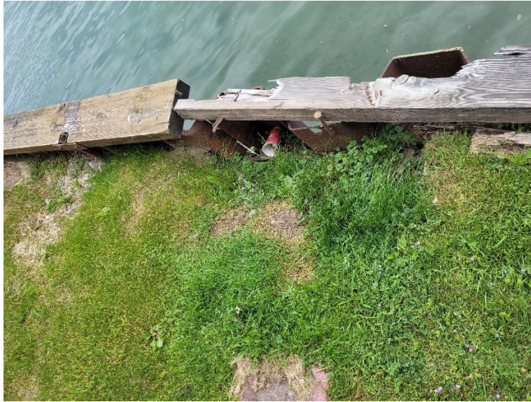
Wood header deterioration
