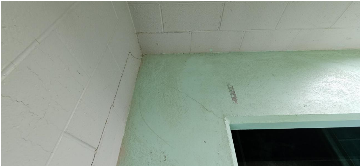
Interior cracking
